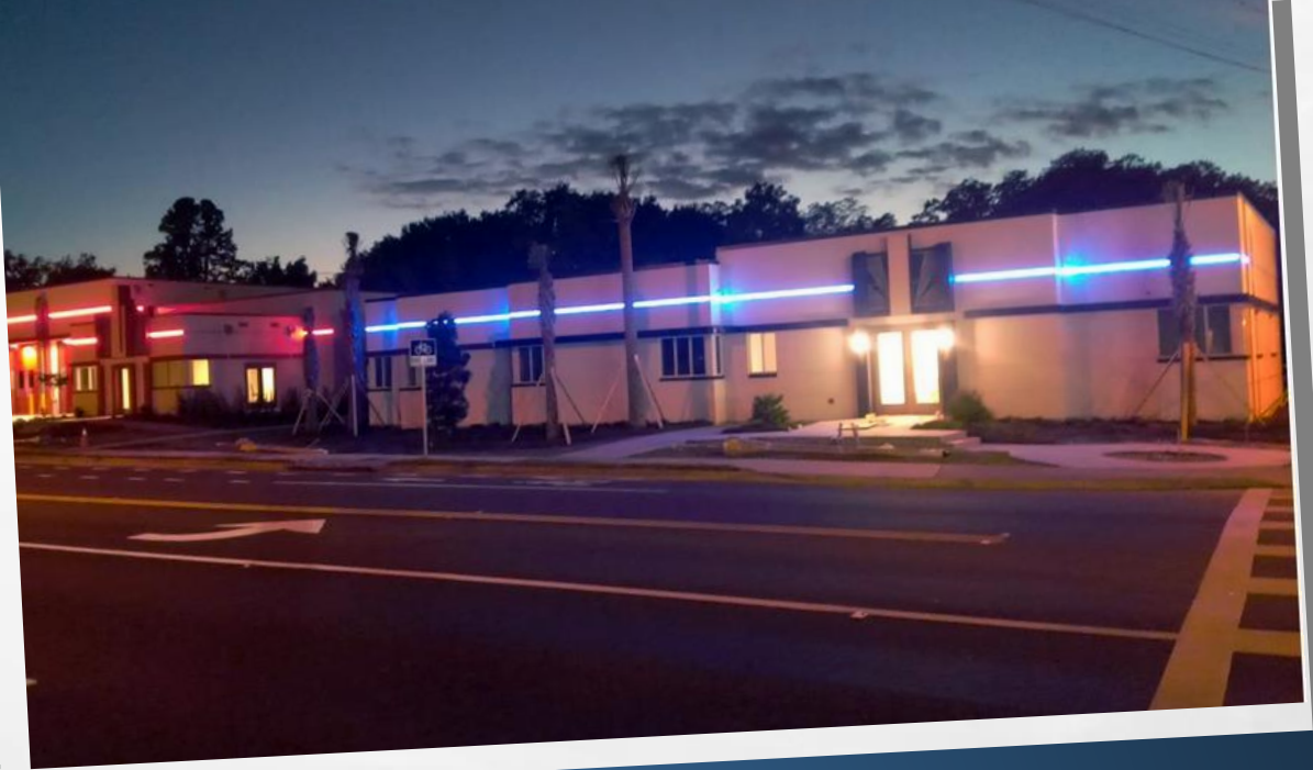
Photo credit to Dinkins Construction
